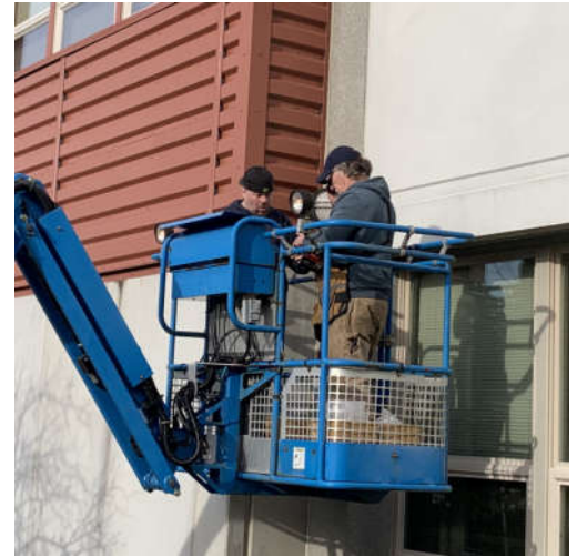
(Right: Dana Wade/Plumber & Donny Sims/Mechanic, assist in replacing light fixtures)
