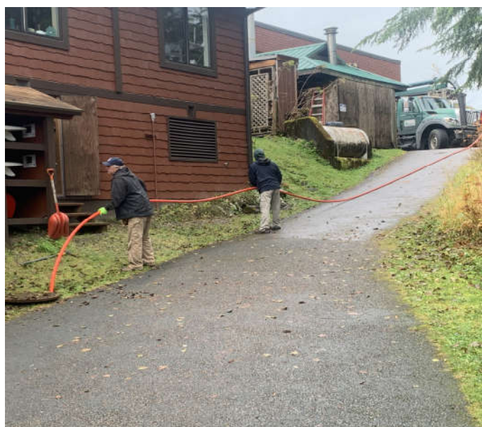
(Left: Dana Wade/Plumber, Bernie Yadao/HVAC pump out clogged sewer line behind the Hendrickson Annex)
