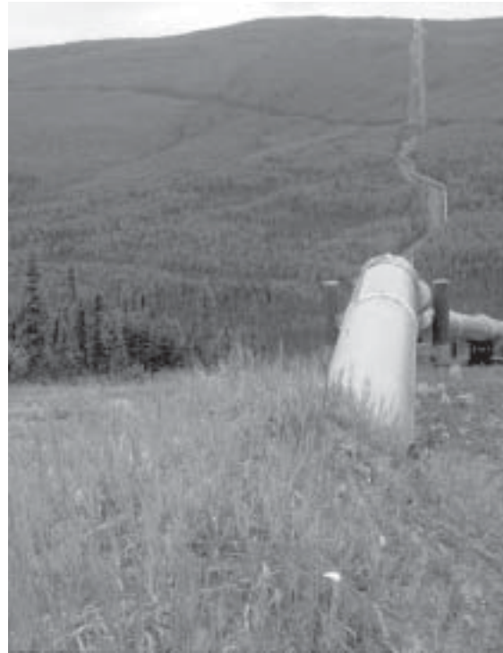
Photo 5. Seeded Bromus inermis growing on mound of soil over buried pipe (MP 396, N65° 29' 26.5"; W148° 41' 17.9'). Survival of this grass species was greatest in this zone of the pipeline corridor. Note the right-of-way has been mowed to control canopy development by woody species, which would otherwise predominate.
