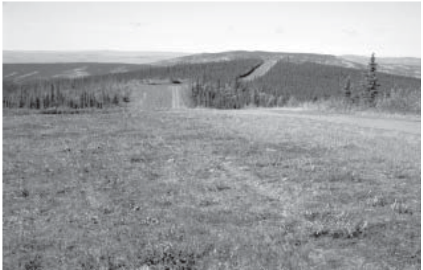
Photo 2. Buried section of TAPS pipeline, north of Fairbanks (N65° 10' 19.3"; W147° 44' 41.2"), with right-of-way recently mowed to remove vegetation canopy. Without repeated mowing, this site would be dominated by brush and trees.
