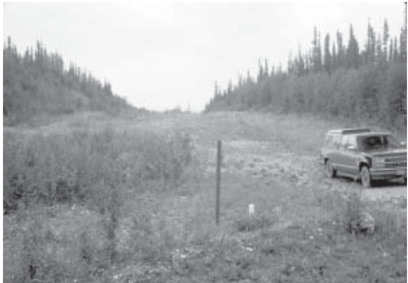
Photo 8. Well-vegetated cut through which the Trans-Alaska Pipeline was buried north of Fairbanks, Alaska. Cut banks on either side of the right-of-way are covered with indigenous shrubs, primarily alder. The central portion of the right-of-way is dominated by a mixture of seeded grasses and indigenous plant species that are growing on the subsoil remaining after construction. In the absence of periodic brushing, the woody species would most likely dominate much of this site. There has been no repeated fertilization of this site. Vegetation is surviving on remaining elements in the original fertilizer applications and natural sources in substrate.
