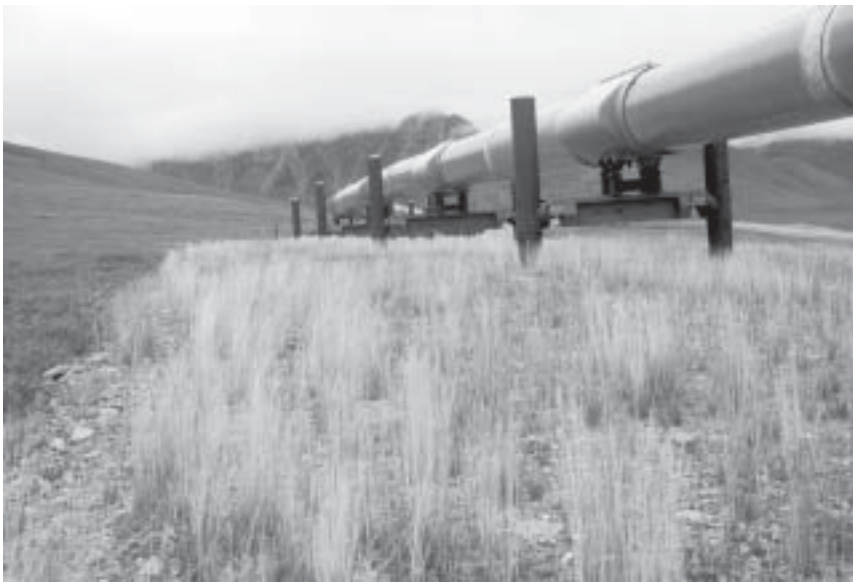
Photo 3. Buried pipeline in northern foothill region of Brooks Range (MP 69, N69° 19' 03.3; W148° 43' 09.7"). Seeded Festuca rubra and naturally established Epilobium latifolium dominate over the pipeline. Naturally colonized Salix alaxensis and Salix lanata var. richardsonii predominate along the margins of the gravel fill and overtop their counterparts in the adjacent undisturbed tundra community.
