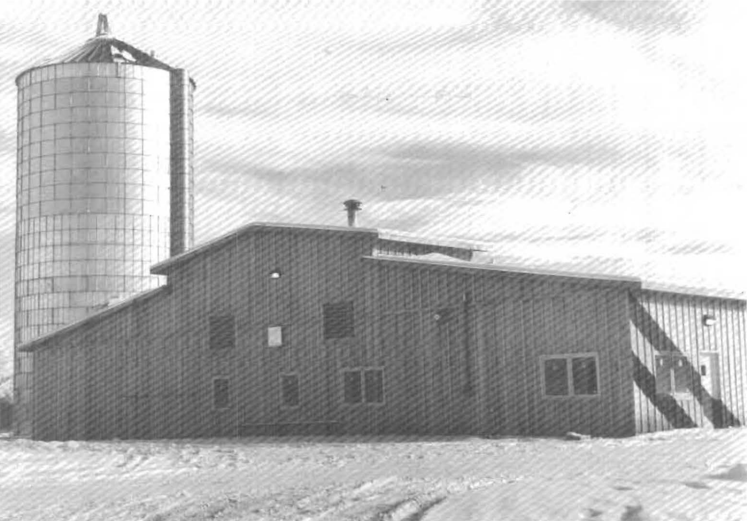
The new barn is constructed of reinforced concrete blocks and has room for 80 cows. Fiberglass insulation is protected by native cottonwood siding. The roof is engineered to withstand 120 m.p.h. winds.
