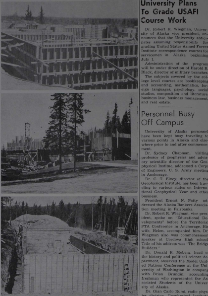
CHANGING CAMPUS —The three photographs above show three more University of Alaska buildings in various stages of construction. At top is the Bonnell Memorial Building, which will be the largest structure on campus and upon which construction will possibly end during the winter of 1959-60. It will replace the old Main Building. In center is the start of another 168-man residence building on campus. The hall which is ready for occupancy this fall. At bottom is the start of a second married students' apartment. Construction will be completed in October or November.
