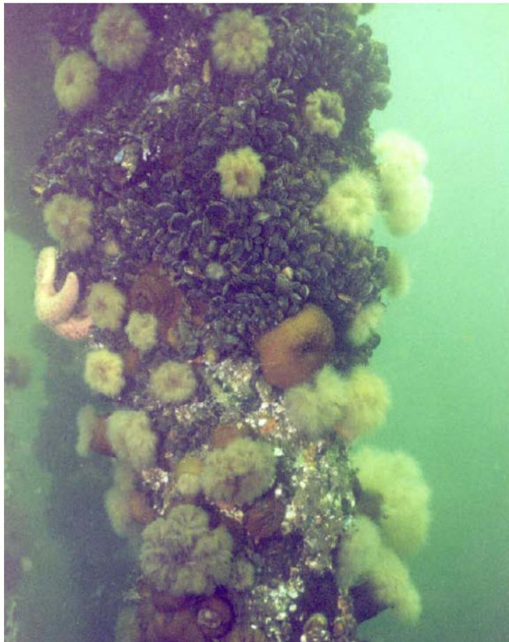
Figure 6.1. Plate 5 from the Sooke Basin study. Marine growth on the BMP piling near the lower end of the mussel (*Mytilus edulis trossulus*) zone (-14' Chart Datum) in October 1999, four years following construction.
