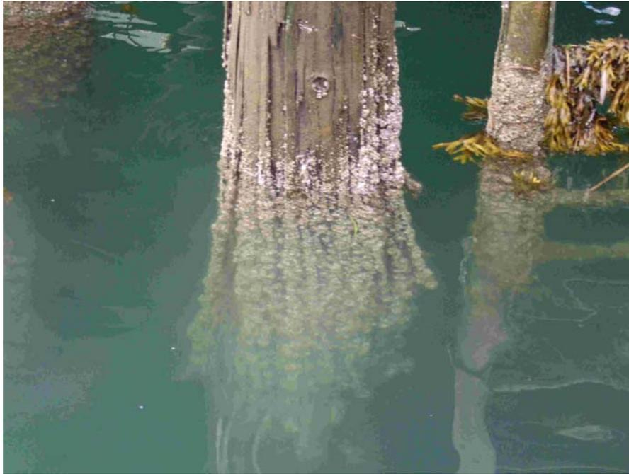
Figure 5.2. An ACZA-treated pile in Juneau, Alaska.
