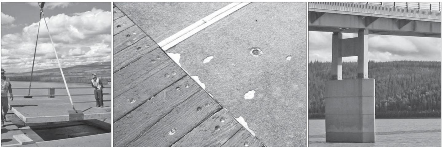
Top right: J. Leroy Hulsey. Photo by Kala Hansen. Bottom Left: AKDOT&PF personnel remove decking from the E.L. Patton Bridge, which crosses the Yukon River. Middle: Close-up of wear to asphalt and wood bridge decking. Both photos by Zach Jerla. Right: Bridge support under the E.L. Patton Bridge. Photo by Mikhail Kanevskiy.
