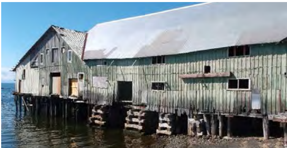
Keku Cannery, Kake. Photo from Alaska Department of Environmental Conservation.
